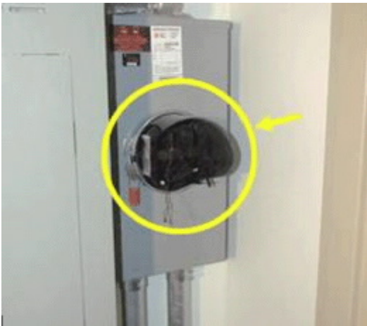
Meter explosion; base plate remained intact
